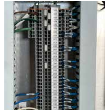
Push-in Terminal Block
