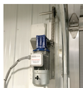
Motor/Jackshaft Assembly
